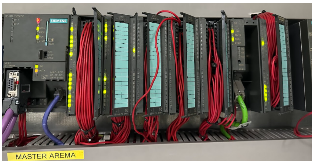
Figura 18. Master Arema - CPU 317-2 PN/DP y TIM3V-IE
