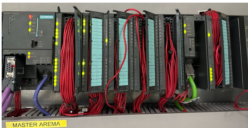
Figura 18. Master Arema - CPU 317-2 PN/DP y TIM3V-IE
